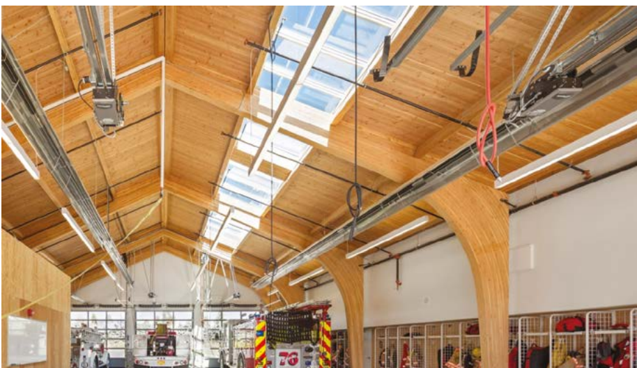
Fire station 76. Oregon, USA. Hennebery Eddy Architects. Fire station built entirely out of wood. Photo: Archdaily.
