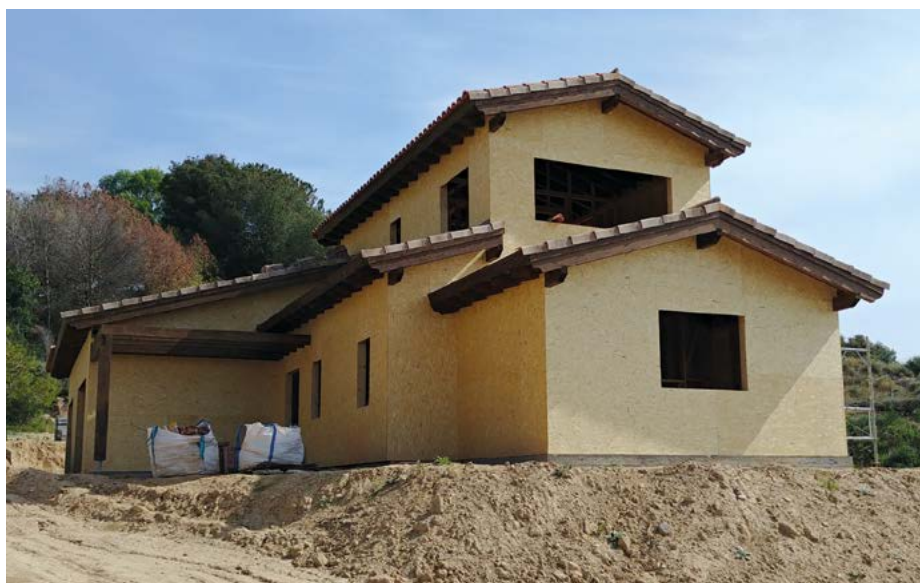
Modern detached house with light frame and OSB panels (Torrefarrera). Photo: Eduard Correal Mòdol. INCAFUST.
