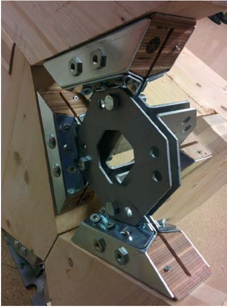
X-RAD system from Rothoblaas, an example of tools for highly complex structural joints for new generation construction solutions with CLT. Photo: Eduard Correal Mòdol. INCAFUST.
