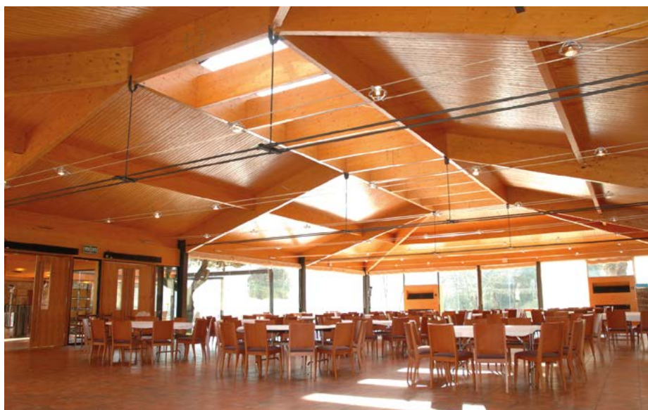
Complex column-free structure built with modern carpentry materials. Photo: Eduard Correal Mòdol. INCAFUST.
