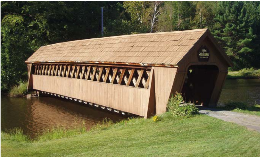
Heavy timber truss bridge (Lincoln, New Hampshire, USA). Photo: Eduard Correal Mòdol. INCAFUST.
