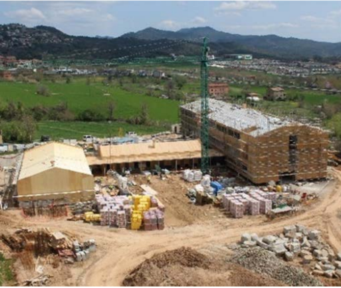
IES Serra Noet - Berga. Photo: Bis Structures.
