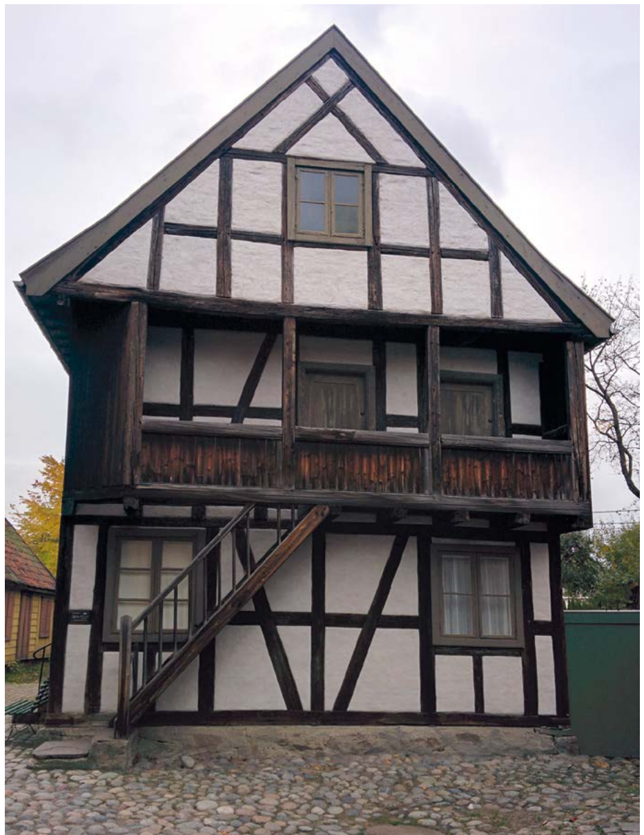
Traditional heavy frame house (Norsk Folkemuseum, Oslo). Photo: Eduard Correal Mòdol. INCAFUST.
