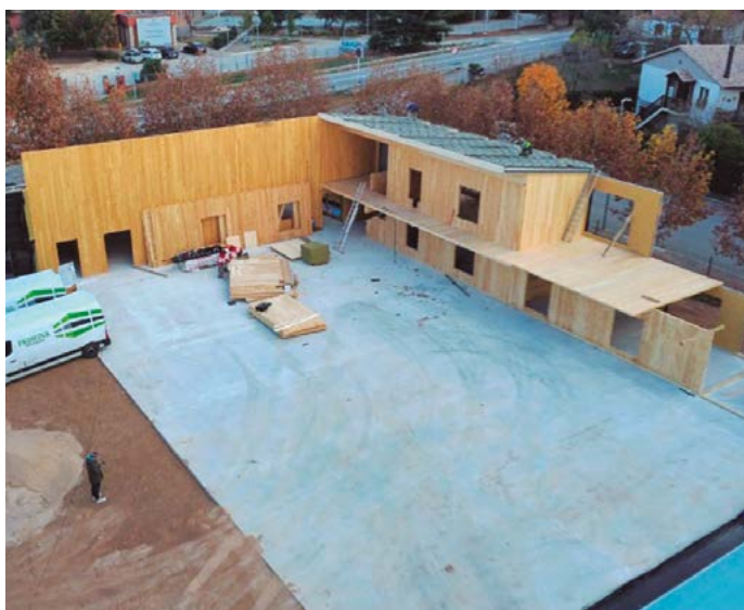
CLT from Catalan wood (forest hub). Photo: Marc Trilla
