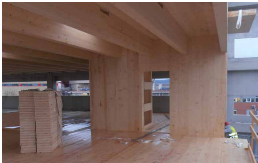
Figura 3: Building constructed with cross-laminated timber.
