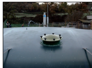
Figura 1: Digestor rural (Font: DAAM, 2010).
